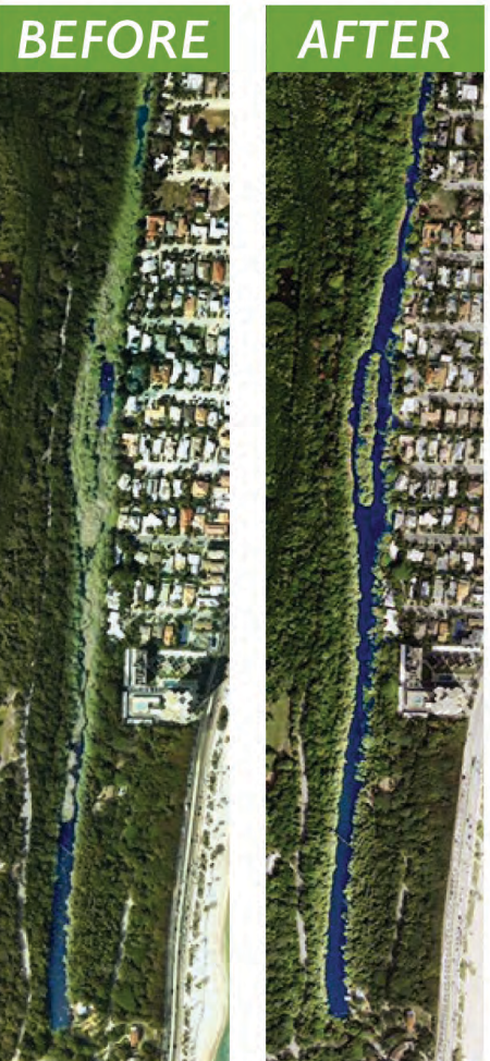
Long Lake Clean-Out Project Phase I completed.
