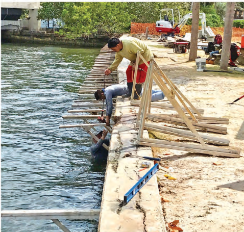
Construction begins on saving the 1.2 mile seawall on the Intracoastal Waterway.
